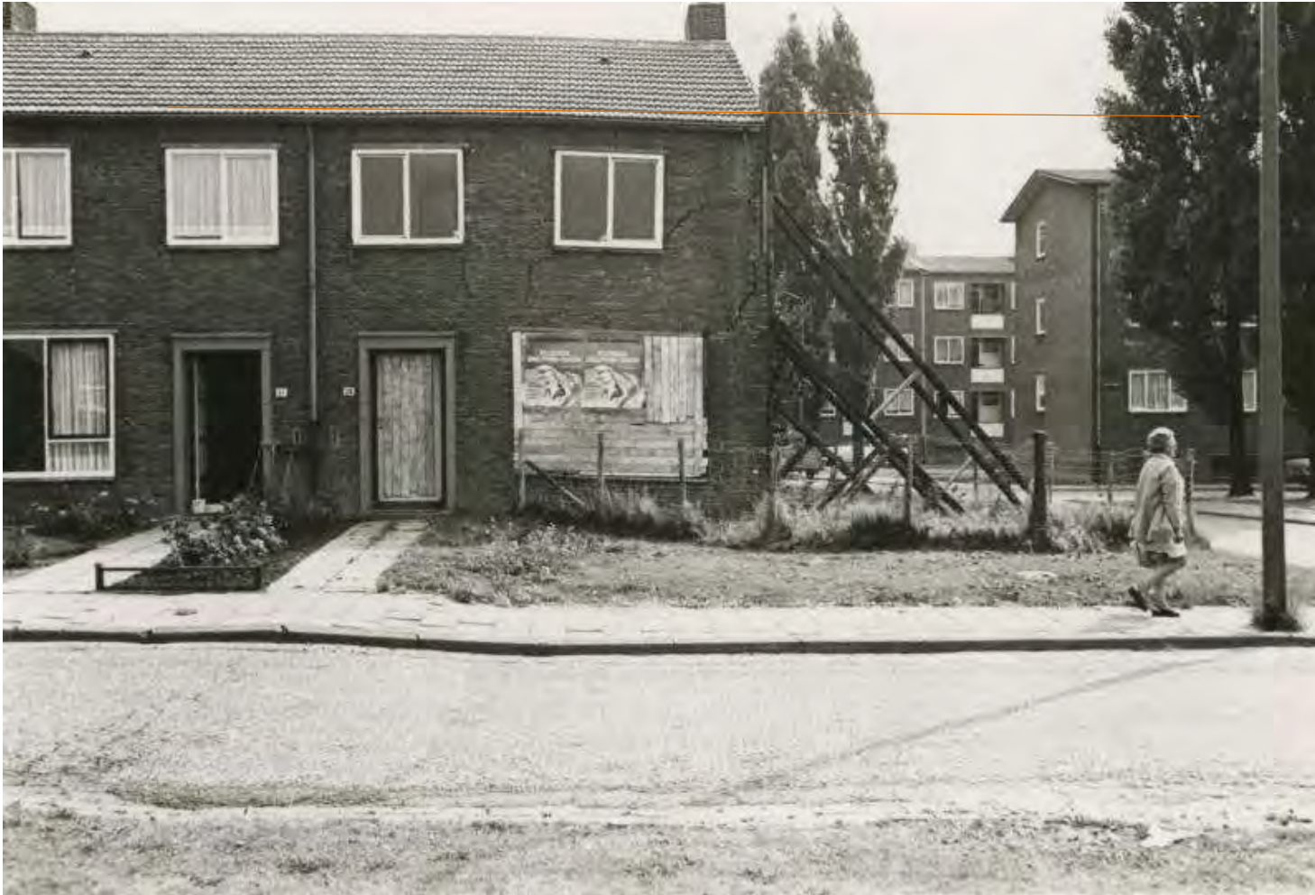
See roof and damage pattern
