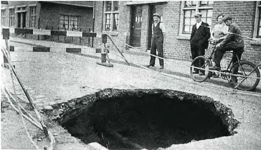
Example of a sinkhole
