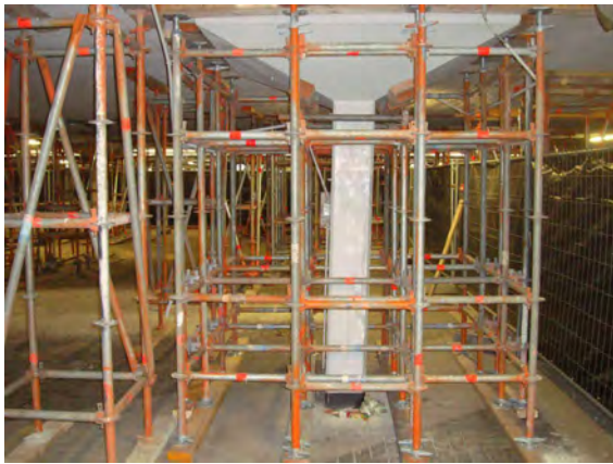
Inclined pillars in garage
