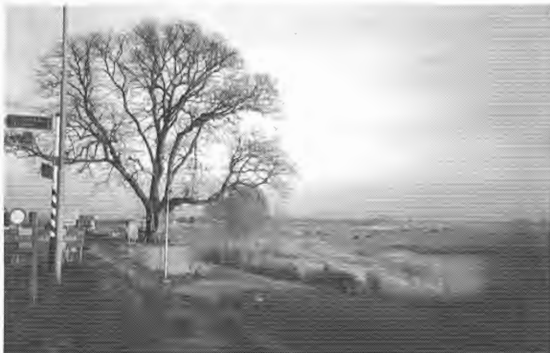
Figure 8 100 year old lime tree near Vuren: a challenge for dike reconstruction. Flood plain ("uiterwaarde" i.e. outer-islet or outer-polder) of the Waal.
