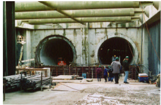
Photo 4. North tunnel portal; TBM already dismantled
