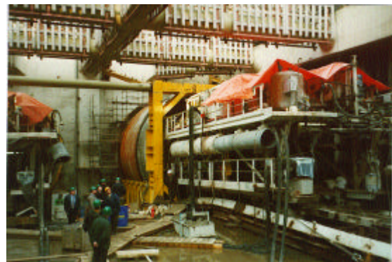
Photo 3. TBM about to start second tube
