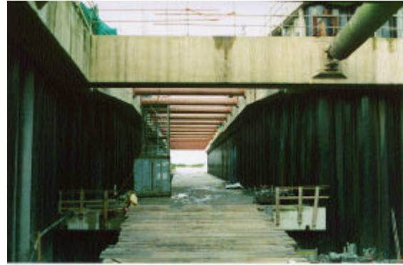
Photo 6. North ramp not yet tractor ready.
