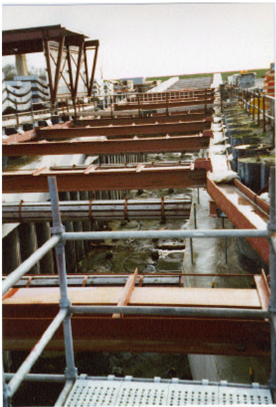
Photo 1. Steel-box frame lifting gear
