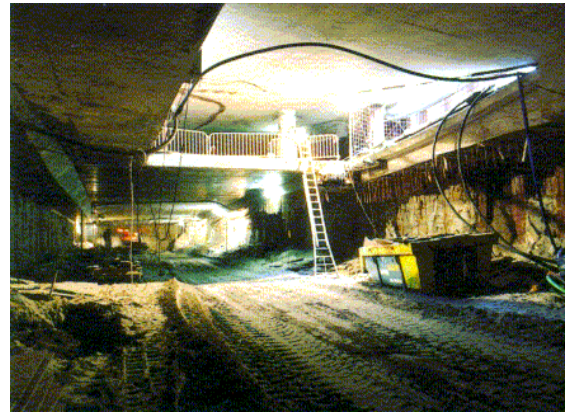
Figure 3. Inside view of the station construction.
