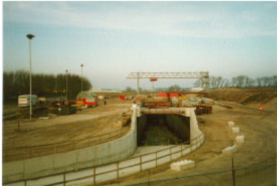
Photo 5. Where tractors and local traffic enters from the south: south ramp
