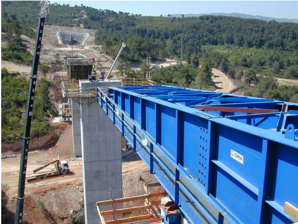
HSL Lilla Bridge
