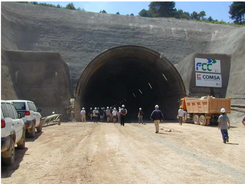
HSL Lilla tunnel portal
