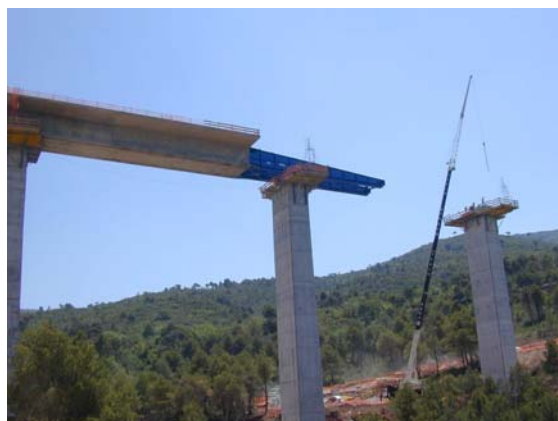
HSL Lilla Bridge
