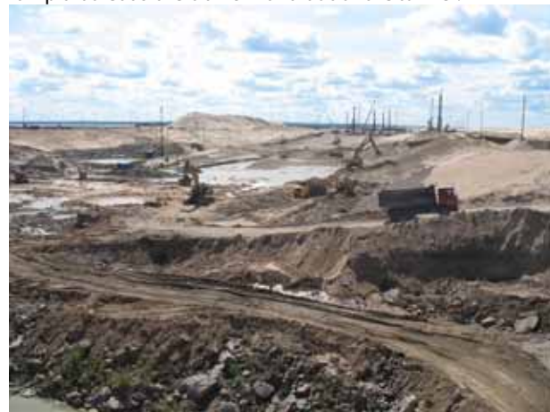
Fig. 6 Excavation of the ramp
