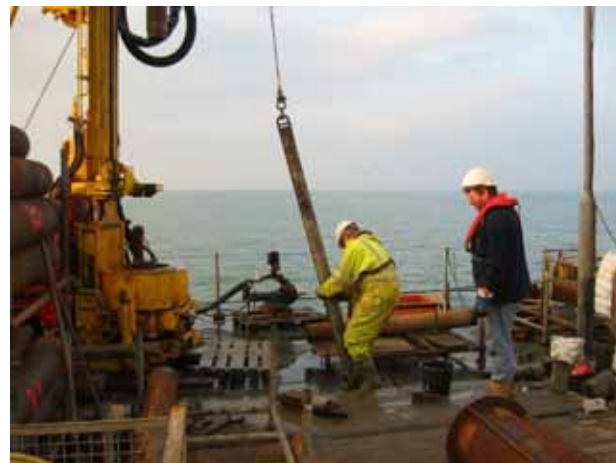
Fig. 4 Drilling activities using a jack-up platform
