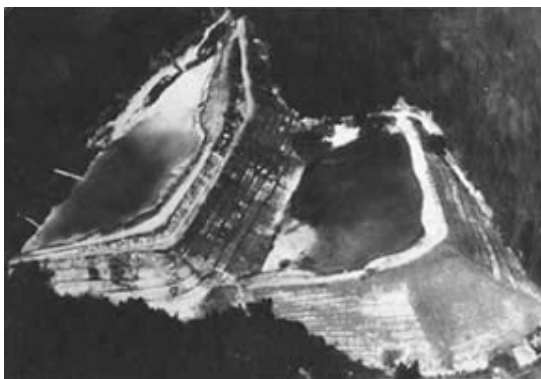
The two settling basins before the disaster. The Prestavel tailings dams were marked by exceptional gradients, unseen elsewhere. (From the newspaper "L'Adige")
