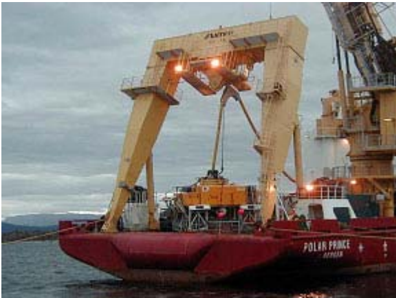
Figure 2. SeaJet ready to be launched from support vessel
