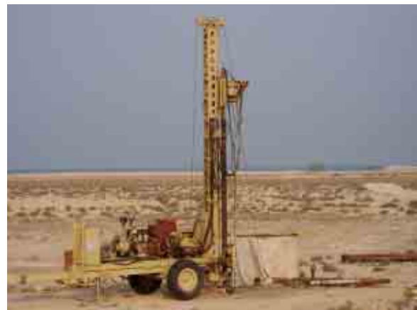
Figure 4: drilling rig in Ras Laffan Industrial City
